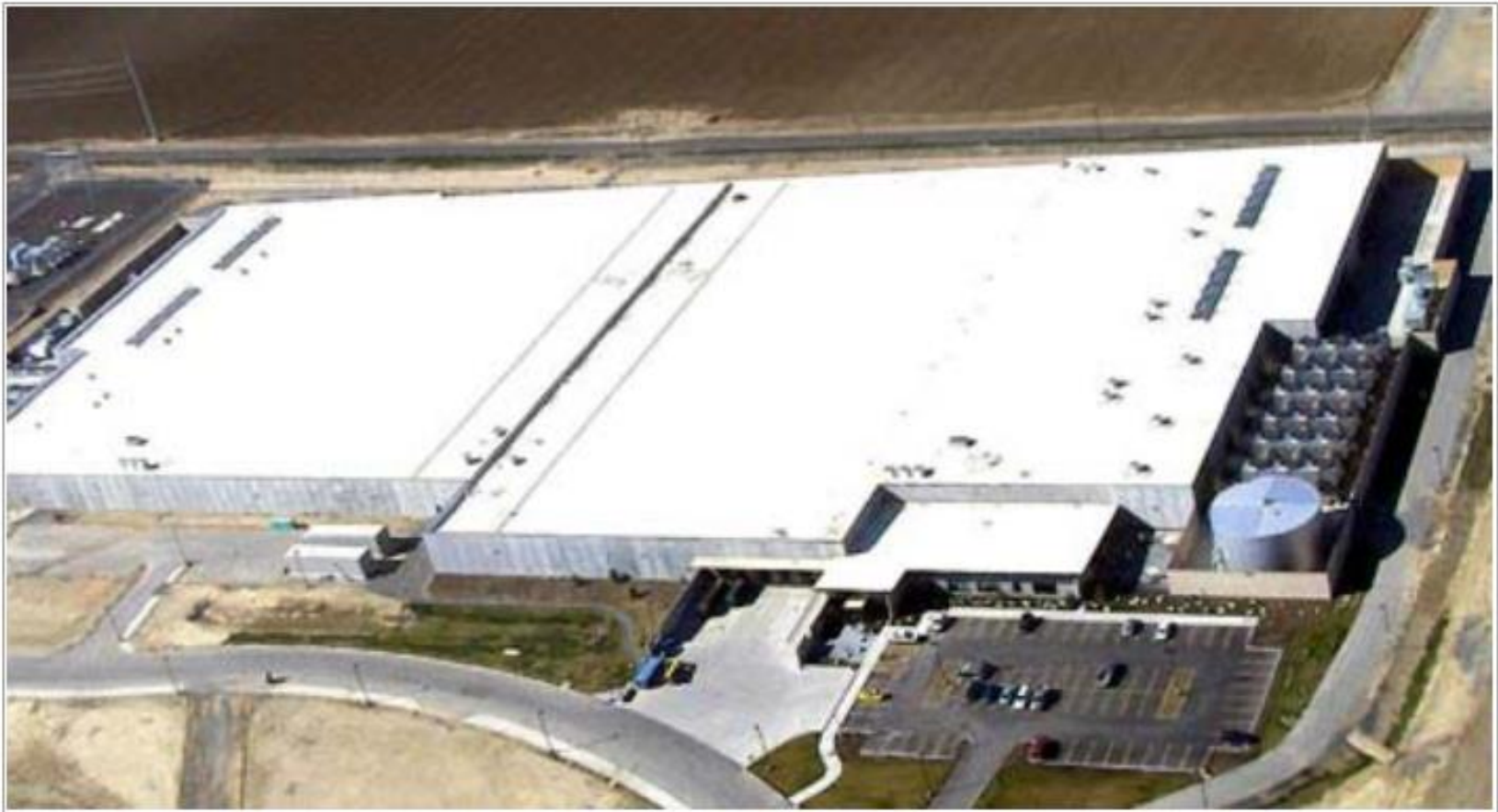
An aerial view of the Microsoft data center in Quincy, Washington
